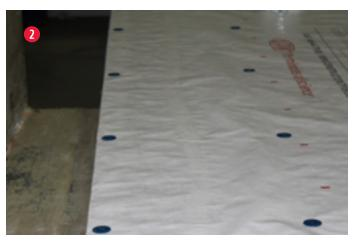
Fasten the DuPont<sup>™</sup> Tyvek<sup>®</sup> WRB to the studs as instructed in the DuPont<sup>™</sup> Tyvek<sup>®</sup> Water-Resistive and Air Barriers Installation Guidelines For Buildings Less Than 5 Stories and Low-Rise Multi-Family Residential Buildings Less Than 6 Stories.
