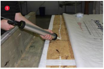
Apply DuPont™ Residential Sealant, or recommended sealant, along the top/bottom of the wall approximately 2 to 3" from the edge. Press the DuPont™ Tyvek® WRB into the sealant using firm hand pressure or a J-roller. This will temporarily hold the Tyvek® WRB in place in prior to step 2.
