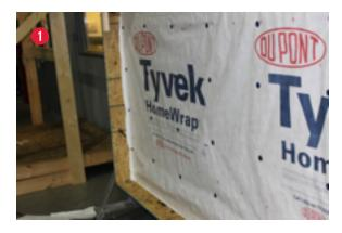
Apply DuPont<sup>™</sup> Residential Sealant or other recommended sealant around the perimeter of the wall framing including the bottom and top plates between the garage and attic.
