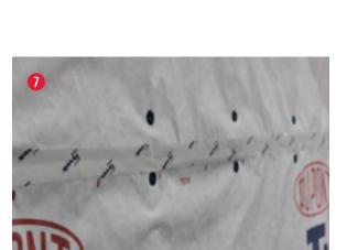
7. Tape all seams with DuPont<sup>™</sup> Tyvek<sup>®</sup> Tape, and verify sealant "connection" between wrap and wood. Use hand pressure or j-roller as necessary to ensure a good bond.
