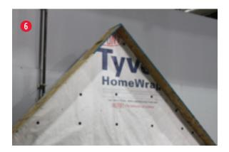
6. Fasten the Tyvek® HomeWrap® as instructed in The DuPont™ Tyvek® Water-Resistive and Air Barriers Installation Guidelines For Buildings Less Than 5 Stories and Low-Rise Multi-Family Residential Buildings Less Than 6 Stories.
