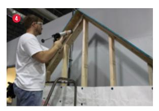
Apply DuPont<sup>™</sup> Residential Sealant or recommended sealant at perimeter of remaining wall framing.
