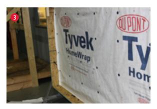
Fasten the DuPont<sup>™</sup> Tyvek<sup>®</sup> WRB as instructed in The DuPont<sup>™</sup> Tyvek<sup>®</sup> Water-Resistive and Air Barriers Installation Guidelines For Buildings Less Than 5 Stories and Low-Rise Multi-Family Residential Buildings Less Than 6 Stories.
