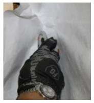
Install the DuPont<sup>™</sup> Tyvek<sup>®</sup> WRB onto framing and tuck edges tightly into sealant and corners of framing as shown above. Use firm hand pressure or J-roller to ensure a positive bond to sealant. Cut excess DuPont<sup>™</sup> Tyvek<sup>®</sup> WRB.
