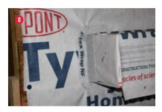
8. Cut another piece (second layer) of DuPont™ FlexWrap™ NF that is at least 12" longer than the height of the cantilever, and install at the corner where the cantilever meets the wall as shown.
