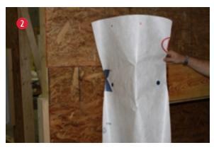
Center the first piece of DuPont<sup>™</sup> Tyvek<sup>®</sup> WRB on the corner of the cantilever and secure with DuPont<sup>™</sup> Tyvek<sup>®</sup> Wrap Caps as shown.
