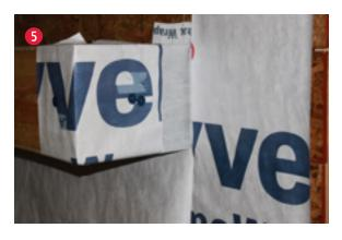
5. Install the DuPont<sup>™</sup> Tyvek<sup>®</sup> WRB starting at the bottom of the wall. When intersecting the bottom surface of the cantilever, create a flap in the DuPont<sup>™</sup> Tyvek<sup>®</sup> WRB by cutting vertically from the top edge to the bottom corners of the cantilever. DuPont<sup>™</sup> Tyvek Wrap Caps or DuPont<sup>™</sup> Tyvek<sup>®</sup> Tape can be used to secure the DuPont<sup>™</sup> Tyvek<sup>®</sup> WRB during this Step.
