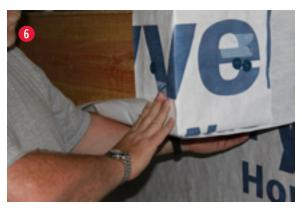
6. Fold flap onto bottom surface and onto face of cantilever as shown, and fasten along the front face of cantilever.
