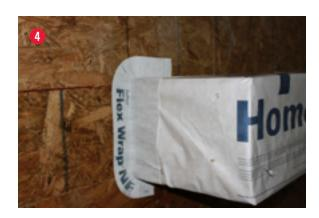
4. Cut a piece of DuPont™ FlexWrap™ NF that is at least 12" longer than the height of the cantilever. Remove the wide piece of release paper and adhere to cantilever surface so it extends 6" onto top and bottom surfaces of the cantilever. Remove second piece of release paper and fan out DuPont™ FlexWrap™ NF onto the face of the wall. Coverage of DuPont™ FlexWrap™ NF should be 2" to 3" onto the face of the wall. Repeat Steps 2-4 on the other end of the cantilever.
