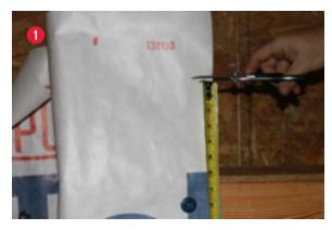
Cut two pieces of DuPont<sup>™</sup> Tyvek<sup>®</sup> WRB that are twice the depth of the cantilever and 12" longer than the height of the cantilever.
