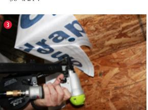
3. Create "package folds" and fasten the HomeWrap® on the top and bottom of the cantilever as shown. Do not install fasteners within 6" from the face of the wall.
