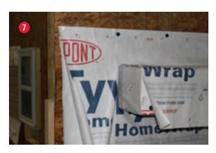
7. Install the next layer of DuPont™ Tyvek® WRB as shown. When intersecting the top surface of the cantilever, create a flap in the DuPont™ Tyvek® WRB by cutting vertically from the bottom edge to the top corners of the cantilever. DuPont™ Tyvek Wrap Caps or DuPont™ Tyvek® Tape can be used to secure the DuPont™ Tyvek® WRB during this Step.
