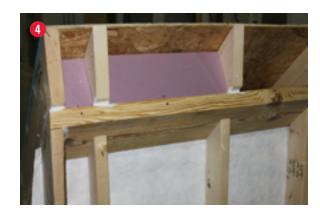
4. Cut ½" expanded polystyrene or equivalent foam blocking to fit openings at rafters and install.
