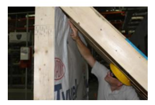
2. Apply DuPont™ Residential Sealant, or recommended sealant, along the top plate and to the remaining 12" of the first and last studs. Install the second layer of the DuPont™ Tyvek® WRB with proper overlap onto the first layer by pressing it into the sealant using firm hand pressure or a J-roller to ensure a good bond between the DuPont™ Tyvek® WRB and the framing.
