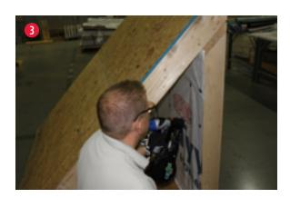
3. Fasten the DuPont<sup>™</sup> Tyvek<sup>®</sup> WRB to the studs as instructed in the DuPont<sup>™</sup> Tyvek<sup>®</sup> Water-Resistive and Air Barriers Installation Guidelines For Buildings Less Than 5 Stories and Low-Rise Multi-Family Residential Buildings Less Than 6 Stories.
