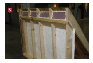
Use DuPont<sup>™</sup> Window & Door Foam to complete seal around foam blocking.
