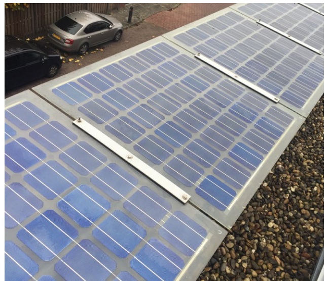
Top: The Donjon's frameless glass panels with clear Tedlar®-based backsheets allow light to pass through.
