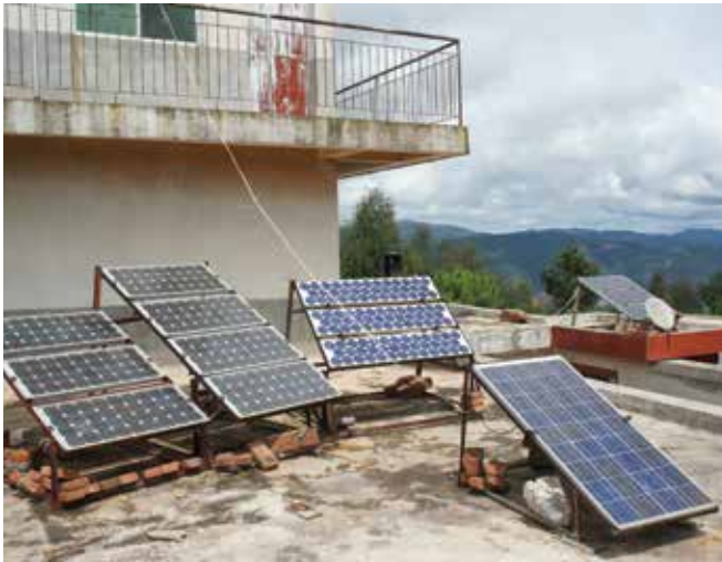
20-year-old panels powering the radar monitoring station at Niuda forest farm, Shiping County, Yunnan Province, China
